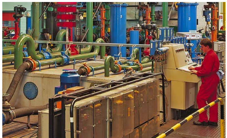
Proefstand SPX Flow Technology in Assen
